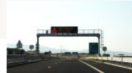
Bulgaria, motorway network
